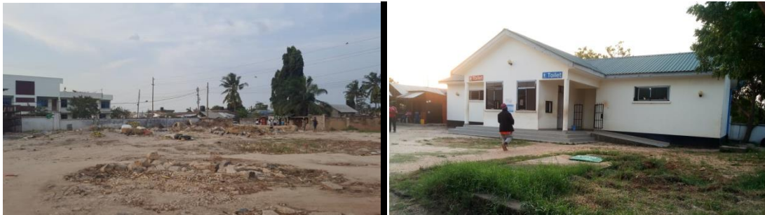
Figure 4: Solid waste collection point and existing Public toilet close to the proposed project site (Source: Field Visit on 25 th July 2021)
